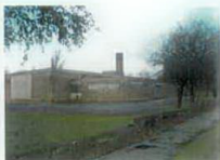
Swimming pool (now removed), looking northeast
